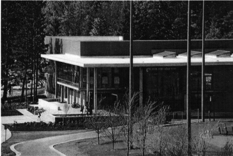
Registered for LEED certification, Wade King Student Recreation Center, WWU. Sustainable Design by Opsis Architecture, Portland © David Scherrer
